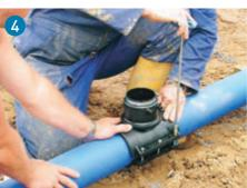
Connection to the plastic pipeline vertically or laterally. Full range of fittings which satisfy all requirements.
