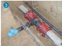
Simple installation technology. PE branch- Tight spaces. POLY16 Plus for easy and off on an asbestos cement pipe with the MULTI/JOINT wide range coupling.
