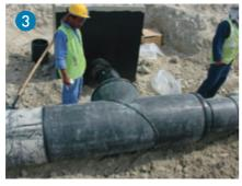
Variety of connection needs. Butt-fused segmented fittings can be customised to meet local requirements.
