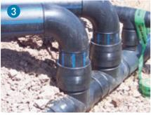
**Electrofusion and spigot fittings up to d630.** Compact and flexible water lines suited to underground conditions.
