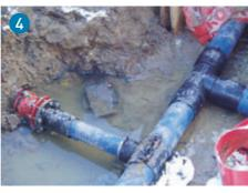
**Wide-range fittings for reliable transitions.** MULTI/JOINT 3000 offers end-load resistance, without thrust blocks.
