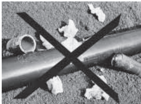
The pipe pit should not be used as a garbage dump
