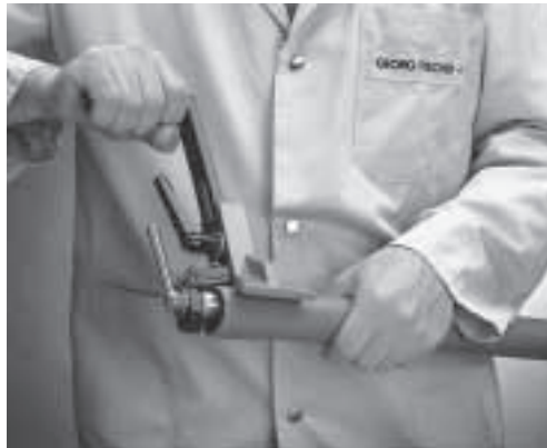
Chamfering the pipe
