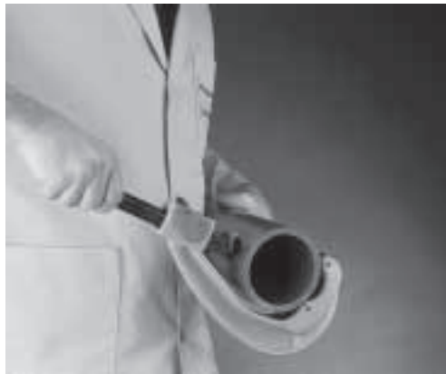
Cutting the pipe to length
