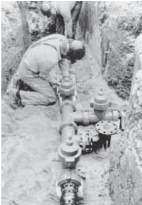
Water distribution with the plastic gate valve system
