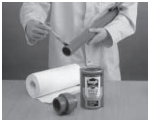
Solvent cement coat at d \leq 90 mm
